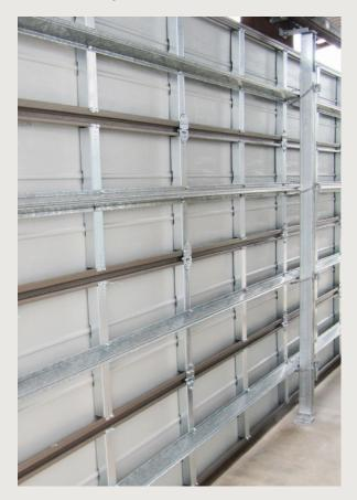
Typical Post to Strut Connection Details
