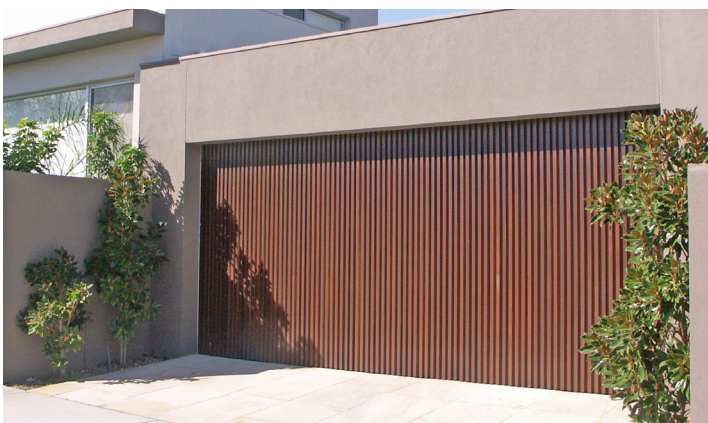
Western Red Cedar Batton onto Plywood Tilt Door
